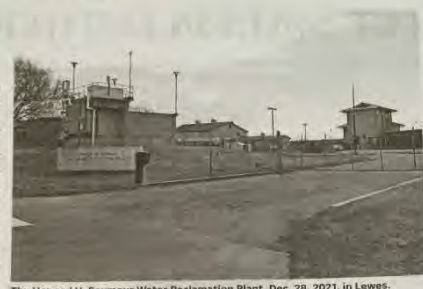
The Howard H. Seymour Water Reclamation Plant, Dec. 28, 2021, in Lewes. LAUREN ROBERTS/SALISBURY DAILY TIMES
